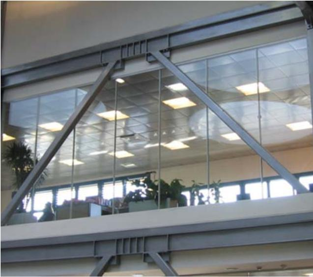
**Figure 1.3** Valorization of internal braces (InterPuls, Reggio Emilia, Italy).
