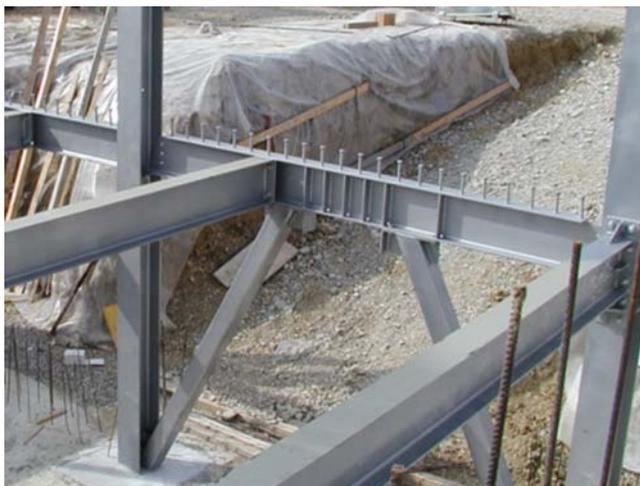
**Figure 4.109** Links in eccentric braces.
